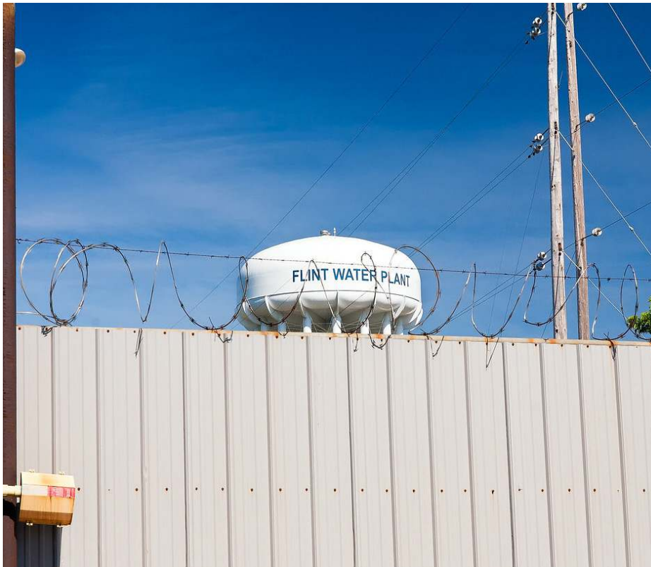
Flint Water Plant, Flint, MI.
