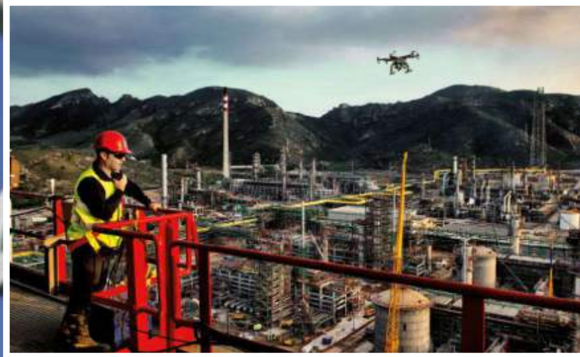
Control de plataformas off-shore (Repsol)
